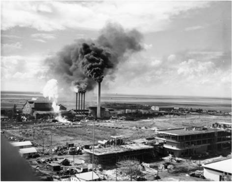
Figure 4.7. By the 1940s, the upper Everglades had been transformed into a highly industrialized landscape. This United States Sugar Corporation refining facility produced a variety of products from cane, including alcohols and synthetic resins. In the foreground is a new “starch house” for processing sweet potatoes for starch for the U.S. war effort. Courtesy of Historical Museum of Southern Florida, Miami News Collection.
