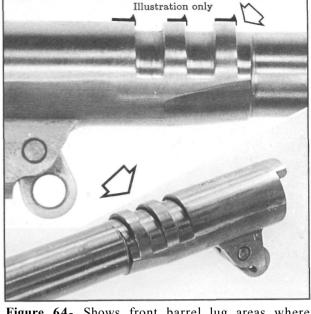
**Figure 64-** Shows front barrel lug areas where lug drag and drag flanging can occur. This condition is mostly found with softer military production [and Colt copy] slides. Colt civilian slides are much better dimensioned and well hardened, virtually eliminating this problem. When dressing, do not lower lugs below .055".
