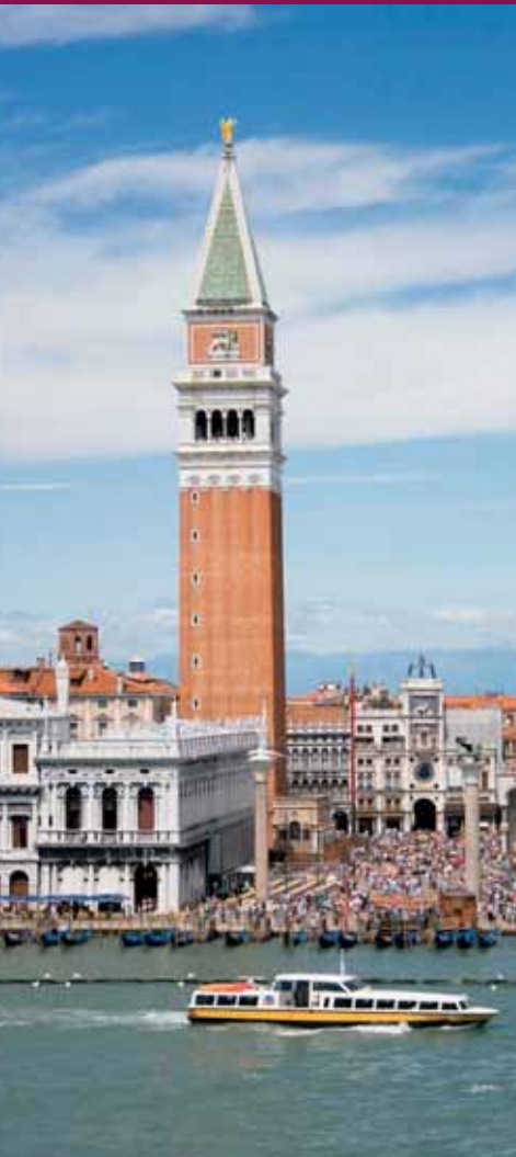
> The 98m (321-ft.) campanile in Piazza San Marco was rebuilt after it collapsed in 1902.
