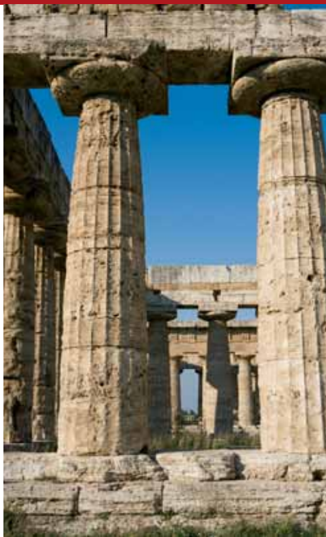
> A classic Doric construction, at Paestum.
