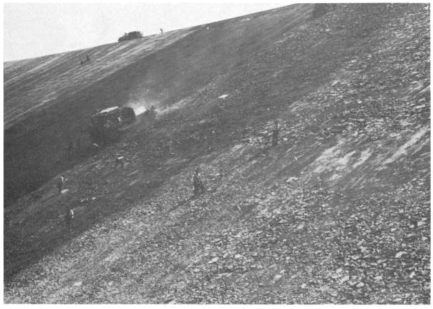
Figure 18.6 Construction of asphaltic membrane: Winscar dam
