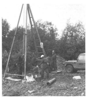
Figure 11.1 Ground investigation using percussion boring equipment on waste tip containing hazardous materials. (*Courtesy*: Wimpey Laboratories Ltd)
