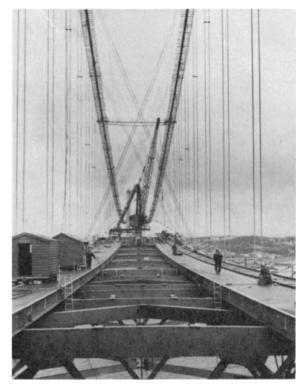
Figure 39.1 This view of the deck of the Forth Road Bridge during erection shows the changes in profile which can occur during the erection process. Arrangements must be made to accommodate and follow such changes in the crane support arrangements. The connections in the structure itself must also accommodate such changes and be designed accordingly
