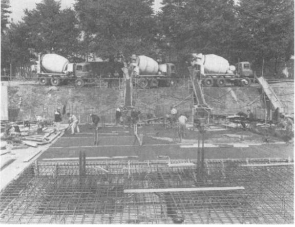
Figure 37.6 Foundation slab being constructed with concrete fed from truck mixers. The concrete is directed down chutes at the side of the excavation. (*Courtesy*: Cement and Concrete Association)
