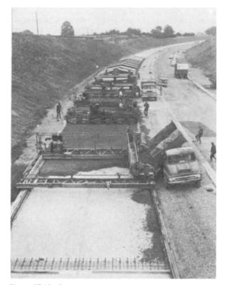
Figure 37.13 Conventional reinforced concrete road construction. Photograph shows from foreground: concrete edge strip carrying rails; sliding membrane and joint assembly; spreading base concrete; laying reinforcement; compacting base concrete through reinforcement; spreading surface concrete; finishing surface with diagonal finishing; texturing and curing (tenting in background)
