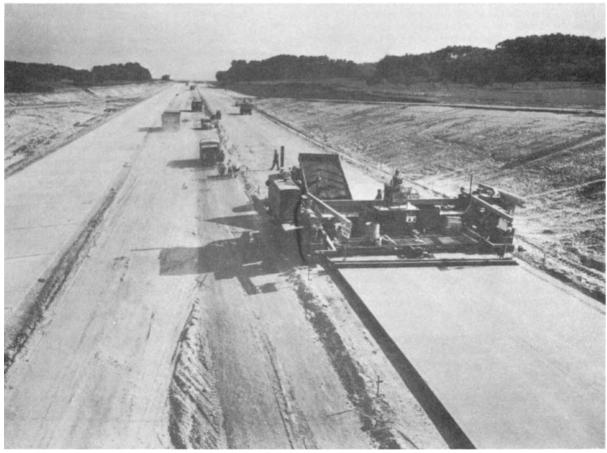
Figure 37.14 Slipform paving with G and Z machine. Unreinforced concrete slab on stabilized base. Transverse joints sawn in hardened concrete of left-hand carriageway after 10 to 24 h
