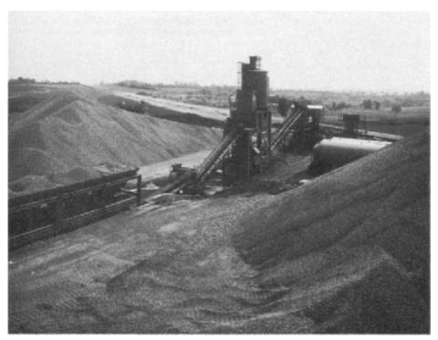
Figure 37.1 Production of concrete for motorway base. *Note*: large aggregate stockpiles; ground storage of cement in wheeled bulk silos; small overhead cement storage; groundwater storage (in background); continuous proportioning and mixing of 4 No. aggregates and cement
