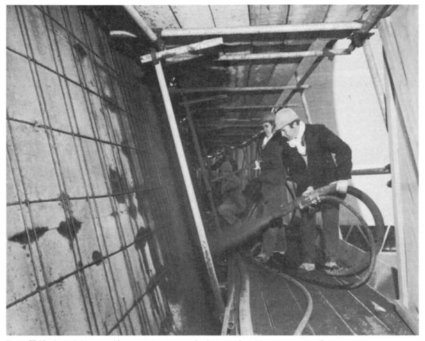
Figure 37.16 Gunite being sprayed from a nozzle to increase the thickness of existing concrete on a cooling tower
