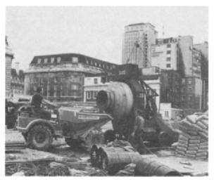
Figure 37.3 Small reversing-drum mixer (Winget 400R). *Note:* drag shovel loading: charge and discharge at opposite ends of the mixer drum; means of controlling point of discharge
