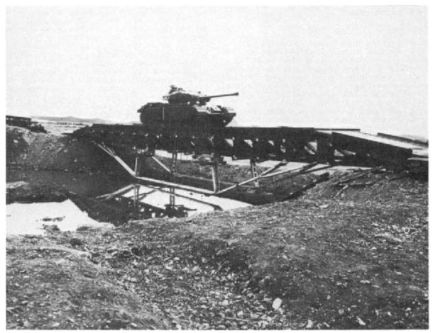
Figure 14.2 Rapidly erectable aluminium bridge for the British Army, built of specially designed extruded sections. The prefabricated units are of welded construction in 7019-T6 alloy. (Crown copyright)
