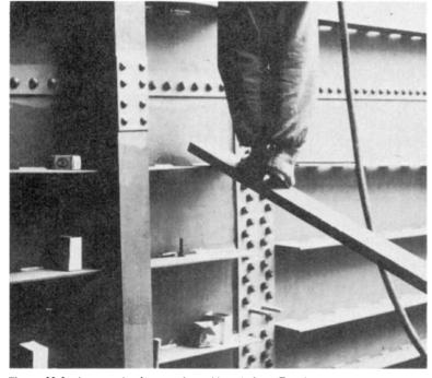
Figure 39.6 An example of an unsafe working platform. To ask a man to work under such conditions endangers not only the man on the platform but also the safety of the other men with whom he is working, and the safety of the whole job could be endangered
