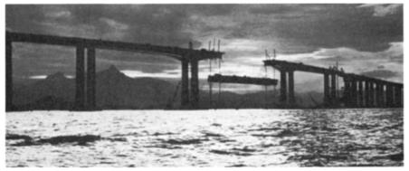
Figure 20.4 Steel girder bridge, Rio-Niteroi, Brazil. (*Courtesy*: Redpath Dorman Long and the Cleveland Bridge and Engineering Co. Ltd)
