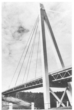
Figure 20.6 Steel trussed cable-stayed bridge. Batman Bridge, Tasmania. (*Courtesy*: Maunsell and Partners)
