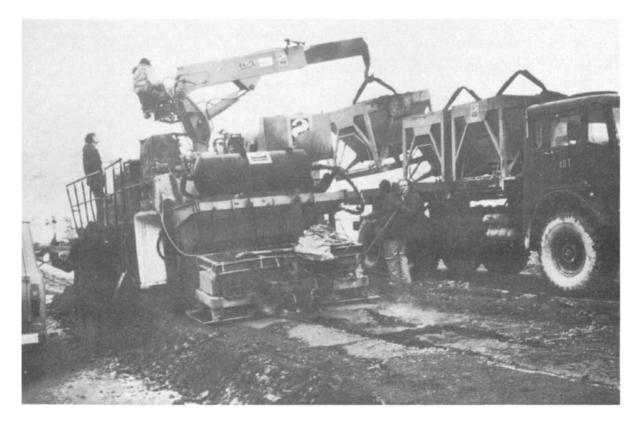
aperture to give the desired width of core and was immediately supported by transition material that had been dumped over the nose. As the machine advanced, guide plates spread the fine granular transition material which was compacted, together with the core leaving, as with the Teerbau machine, a firm level surface to the 200 to 250 mm lift of core plus transition.
