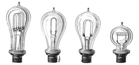
FIGURE 2.4. Different kinds of Edison's light bulbs from the 1880s. Reproduced from Figuier (1888).
